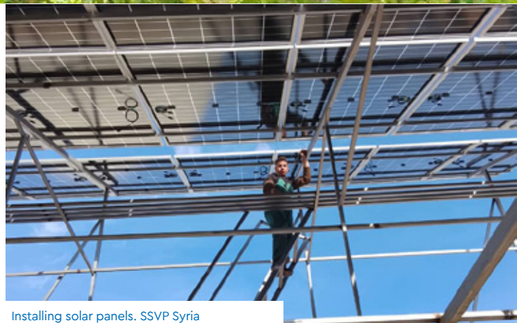
Installing solar panels. SSVP Syria
