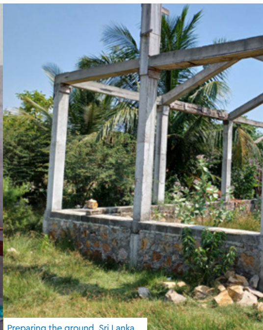
Preparing the ground, Sri Lanka
